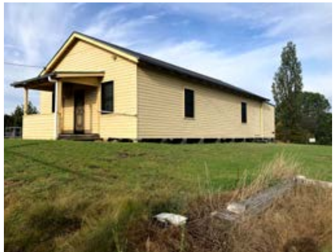
Photo 5: Existing band hall building (to be removed). Pump track to be located on / behind the building's current location.
